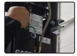
Hold the system by the hand cutouts, carefully hang the frame on the channel strut. Ensure both tabs on the frame are secured between the bolt heads and channel strut.
