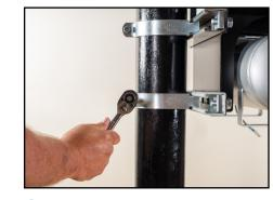
Slide the second set of pipe clamps into the bottom channel strut already attached to the system. Secure clamp bolt & nut. (Adjustable wrench and 9/16 wrenchl
