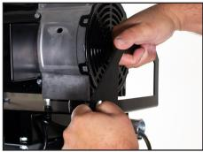
CAUTION: THIS IS A TWO PERSON LIFT. Hold the system by the hand cutouts, carefully hang the frame on the channel strut. Ensure both tabs on the frame are secured between the holt heads and channel strut.
