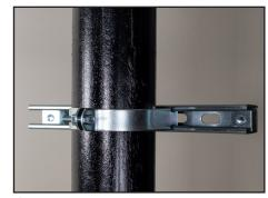
Use the included (shipped loose) top channel strut, install using the proper sized clamps for the riser pipe diameter. A kit of clamps is included with every unit. Make sure the top strut channel is level and secure clamp bolt & nut.
